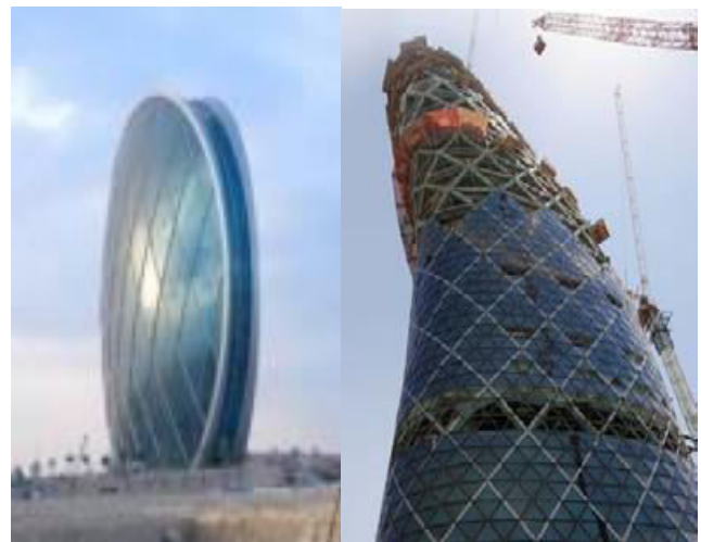
Fig -9 Al Dar Headquarters Fig -10 Capital Gate (Images source: Sepideh Korsavi & Mohammad Reza Maqhareh-2014)
