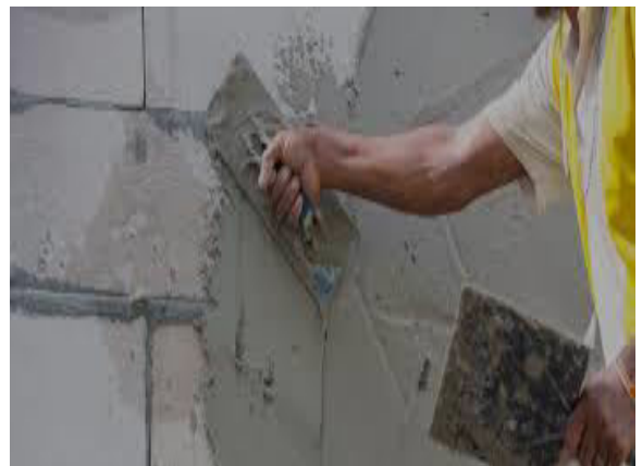
Fig -6 Wall plastering to avoid seepage
