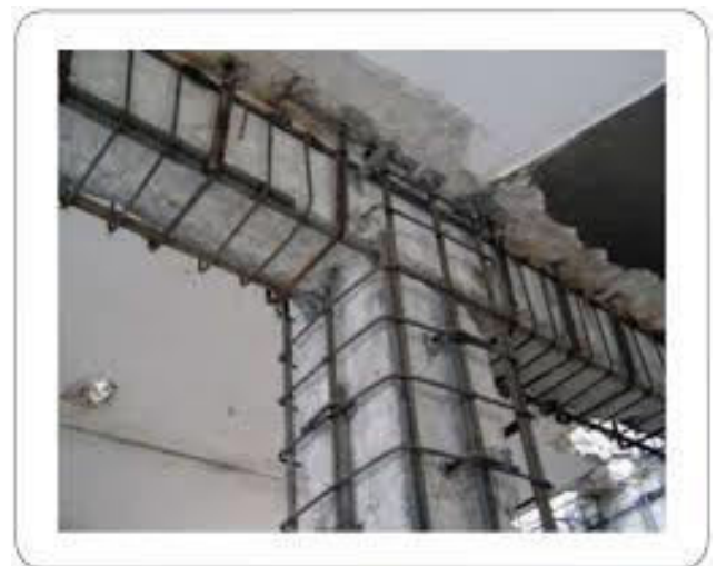
Fig -7 Column and beam jacketing
