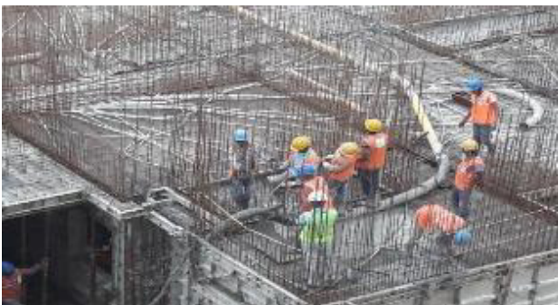
Figure 4 :Concrete Pouring work
