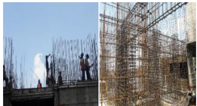
Figure 2 :Shear Reinforcement
