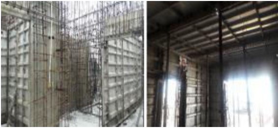
Figure 3 :Erection of Formwork shuttering
