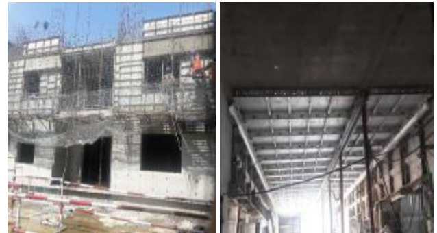
Figure 5 :Striking of Mivan Formwork
