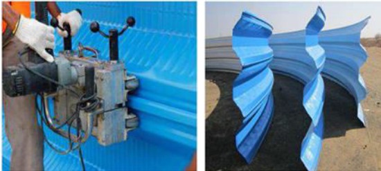
Fig.3 Mechanical Seaming & Grouping of three members at Ground
