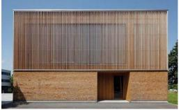
Figure 3.1.1: Building having Opaque material façade restricting light from entering.
