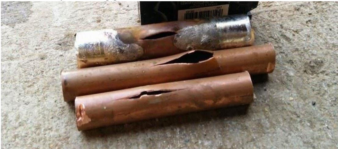
Figure 9 Drill pipe failure, Burst
