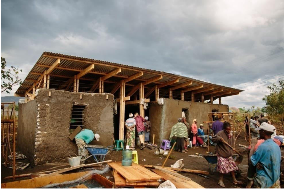
Figure 3: Sandbag House Construction process
