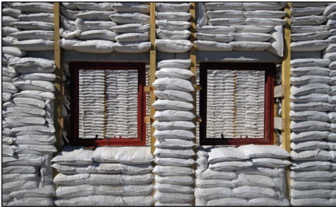
Figure 2: Construction Phase of 10 X 10 Design Indaba, Low Cost-Sandbag Homes
