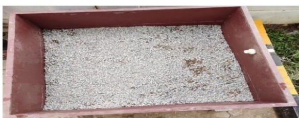
Fig7.1.4: Filled with 6mm aggregates .
