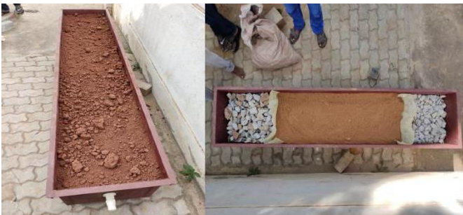
Fig7.2.4 & 7.2.5 : Showing inlet and outlet Portion 40mm aggregates, middle portion filling fine aggregates
