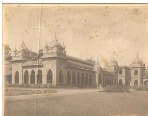
Fig -7: SSG Hospital
