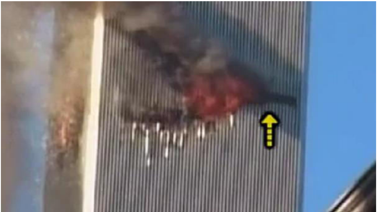
Structural damage and set off intense fire after crashing
