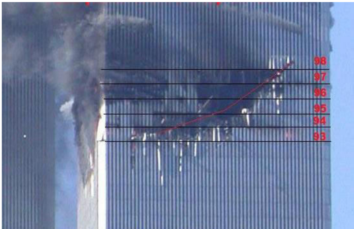
Impact zone lost the ability to support above load
