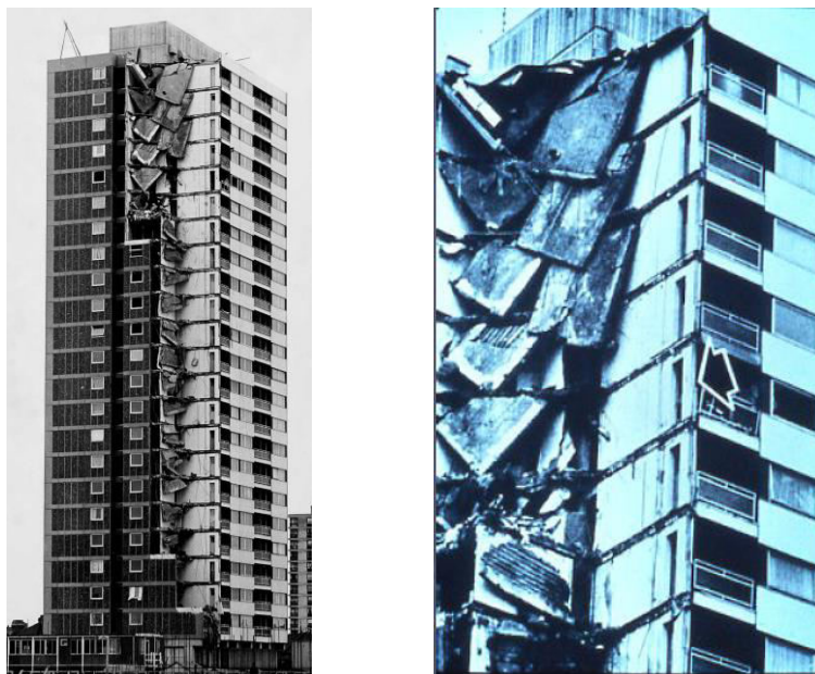
Fig.1.2 Ronan Point, 1968 –Collapse due to gas explosion
