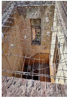
Figure 6 Deteriorated and destructed slab
