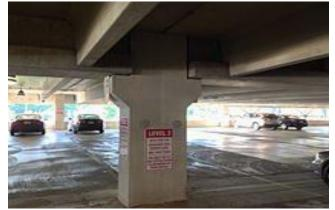
Fig 1.Precast parking structure showing an interior column, girders, and double-tee structural floors. The two gray circles are covers to close the lifting anchor holes.
