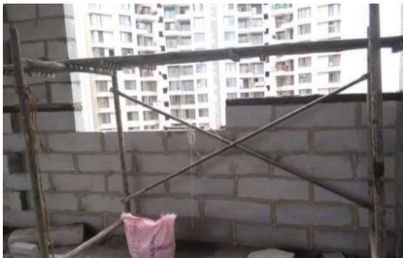
Fig -4: Placing of block
