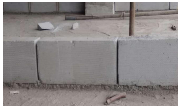
Fig -2: Laying of block
