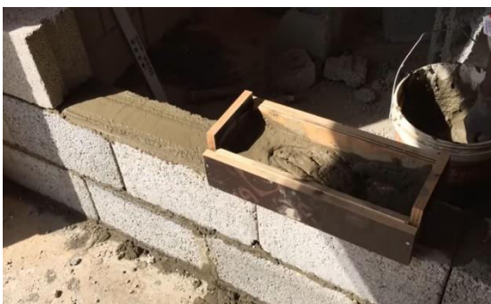
Fig -5: Laying Mortar by using Optimization technique
