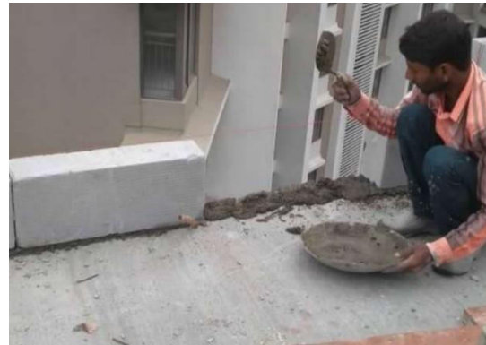
Fig -1: Laying ground mortar
