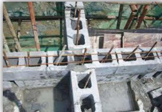
All the walls in house are built with hollow blocks and filled with concrete. Block is a mix of concrete and wood which acts and anti-bacterial and has great insulation properties. Insulation is provided inside the blocks to prevent energy loss. Hollow blocks are used to make walls that handles moisture and insulates at the same time, the blocks are filled with concrete (which is having 50 % fly ash replacement for the Portland cement) and smaller rebar's
