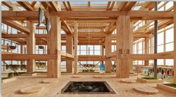
Zero energy house uses glue laminated timber (which has low carbon footprint) as the main structural element in place of concrete and steel, so reduces the overall weight of the structure and also less damage in case of any natural disasters.
