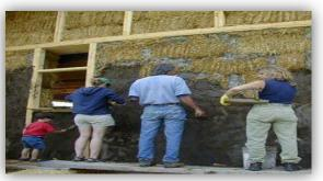
To maintain the comfortable humidity inside the house the walls are plastered with a **special plaster which is a green material,** and it has the capacity to absorb the moisture from air giving a maintained humidity inside the house. The cooling system is also used as dehumidifying machine, in case we want to reduce the relative humidity of house, the variable speed fan starts sending lesser air thru blowers further into the house which results to low humidity.
