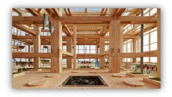
Zero energy house uses glue laminated timber (which has low carbon footprint) as the main structural element in place of concrete and steel, so reduces the overall weight of the structure and also less damage in case of any natural disasters.
