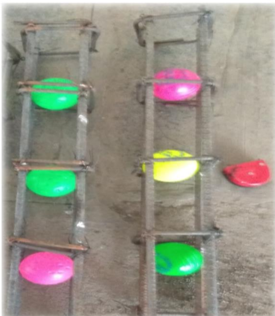
Fig. 2.1: Beam Reinforcement (hollow bubbles)
