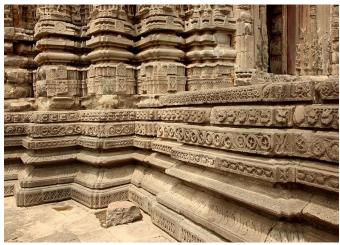
Fig -8: Typical molding plinths of Yadava temple
