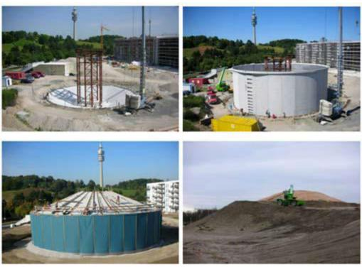
Figure 2 Construction of a tank thermal energy storage system [17]
