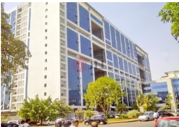
Fig 2 North west Facade
