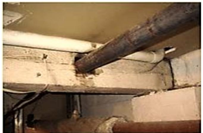
**Figure 1:** Illustration of utility openings integrated within RC beams in a real-world building scenario [14].
