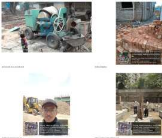
Fig. 1. Selected construction-site activities documented during industrial training.
