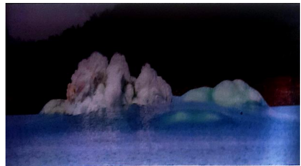
Figure 2 Lake tapping at koyna hydro project
