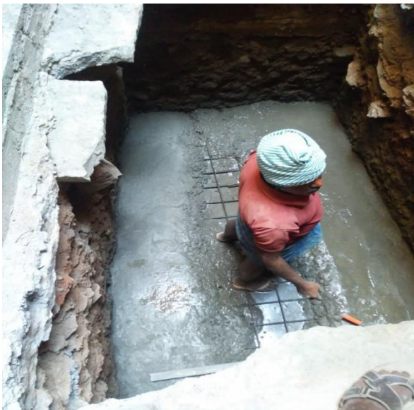
Fig no: 6.1 Concrete poured in rebar placement
