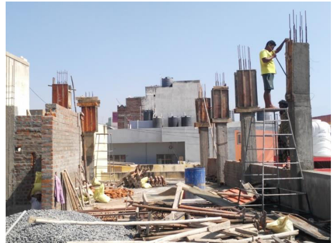
Fig no: 5.1 Formwork for Column
