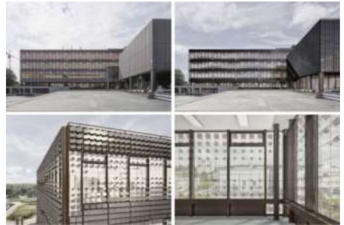
Fig -1: The Adaptive Solar Facade (ASF) retrofitted on the HIL building at ETH Zürich.
