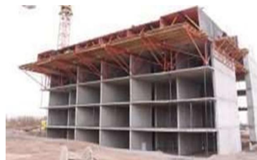
Fig. No. 7 Tunnel Formwork System
