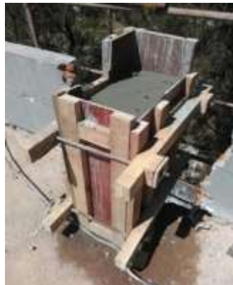
Fig. 4. Concreting with micro concrete
