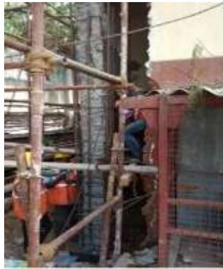
Fig. 2. Additional Reinforcement
