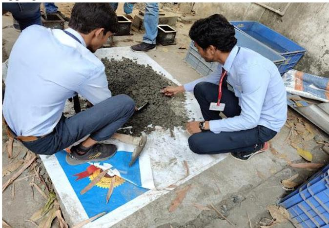
Fig-1: Mixing of Concrete
