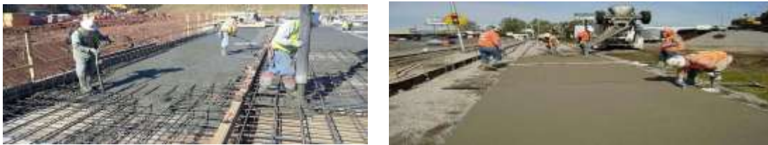
Fig 1. Road Grading construction
