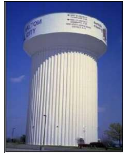
Figure 1: Overhead Water Tank
