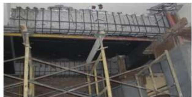
Figure 6 Jacketing of Beam
