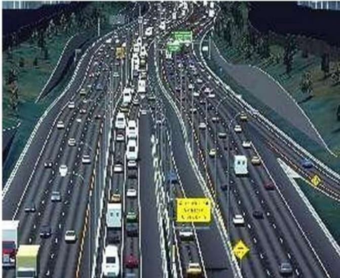
Fig -1: Concept drawing of an Automated Highway System with dedicated lanes in the center of the highway.
