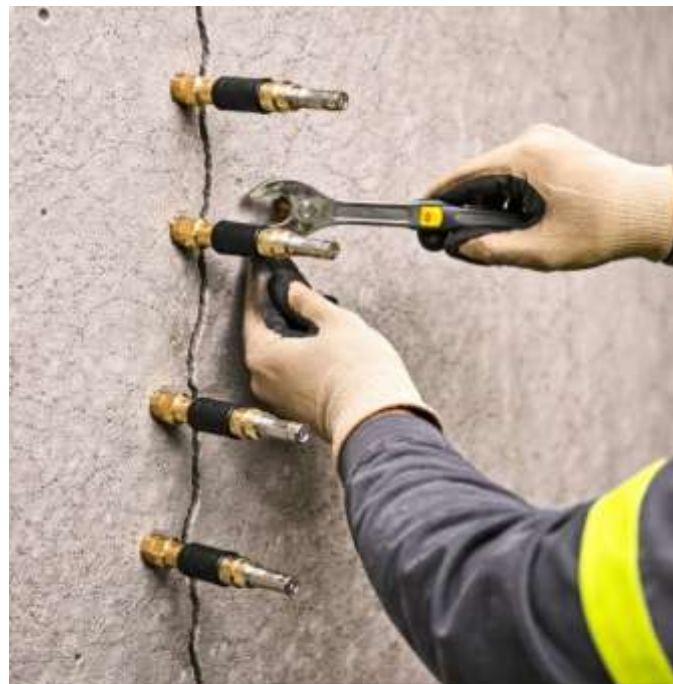
Installation of Nozzle Packers
