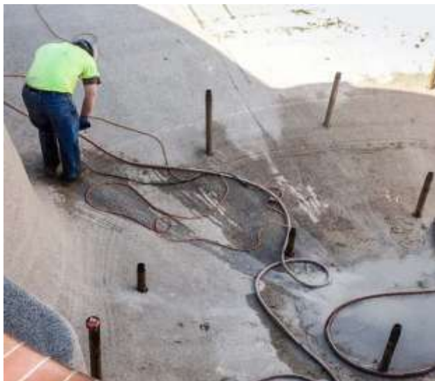
Figure 9 Inject Grouting
