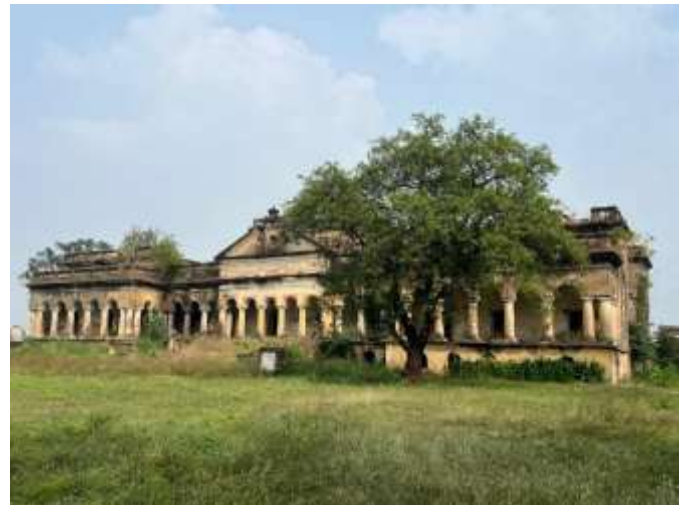
Fig -1: Laxmipur palace, Laxmipur village, Panna, Madhya Pradesh; Source: Author
