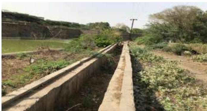
FIGURE : 16 CONSTRUCTION OF DRAIN
