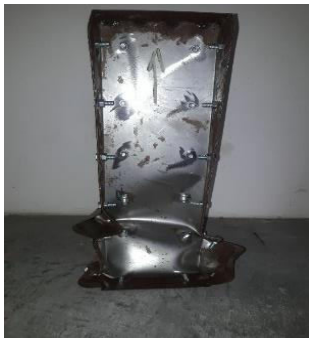
Fig 13: Failure of bolted column
