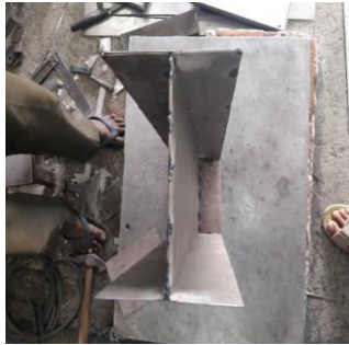
Fig 6: Welded connection at web
