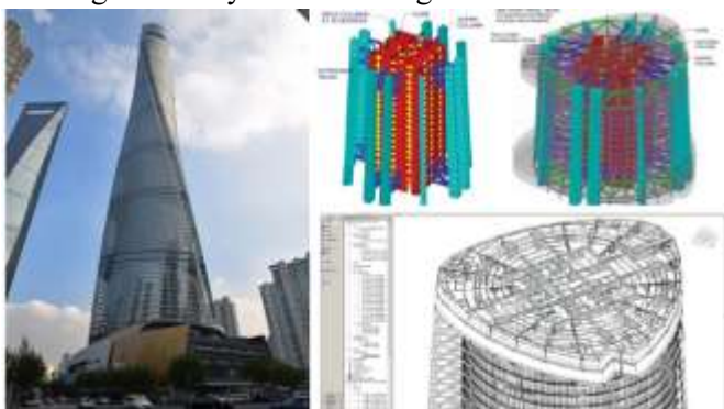
Fig -14: BIM and structural models of Shanghai Tower
