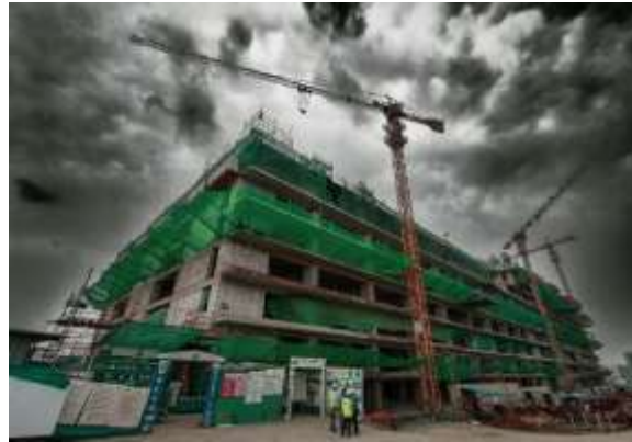
Fig.4.1.2. During construction phase
