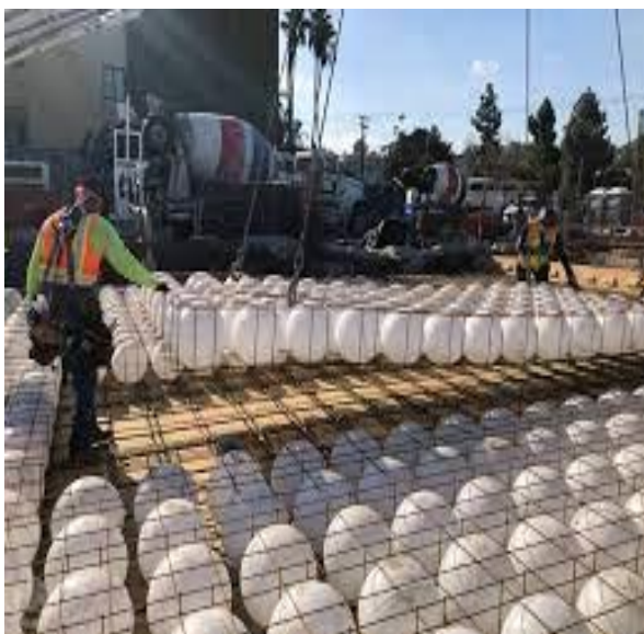
Fig. 2. Process of bubble deck slab
