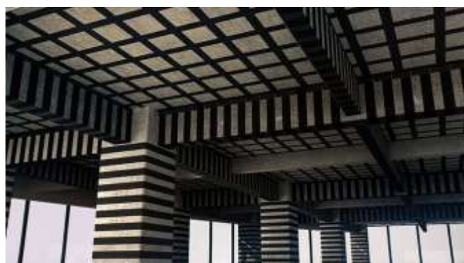
Figure 7. CFRP Works in Retrofitting
