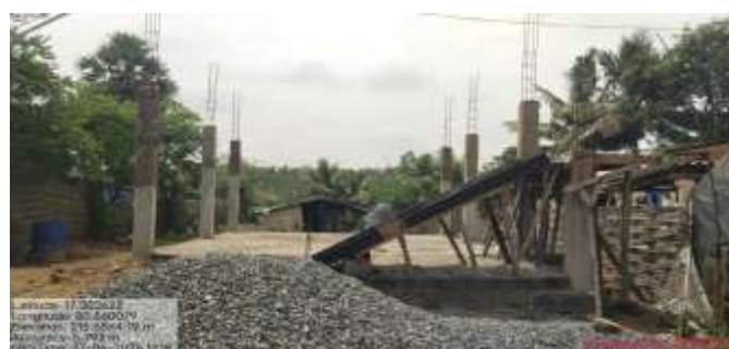
New Demo House Stage -1
