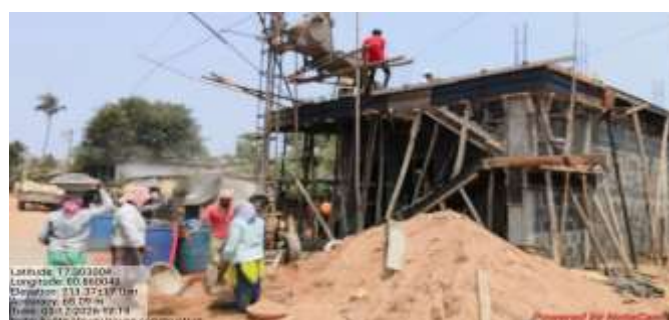
Demo House Slab Casting - 2
