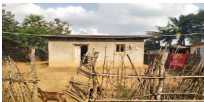
Figure 5. Representative external view of a surveyed IAY house, showing the single-storey load-bearing masonry construction typical of the cluster.
