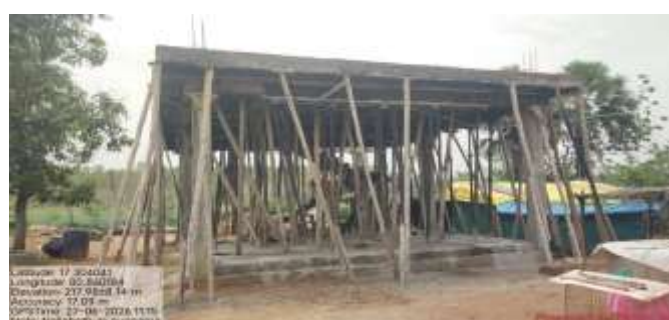
Demo House Slab Completion
