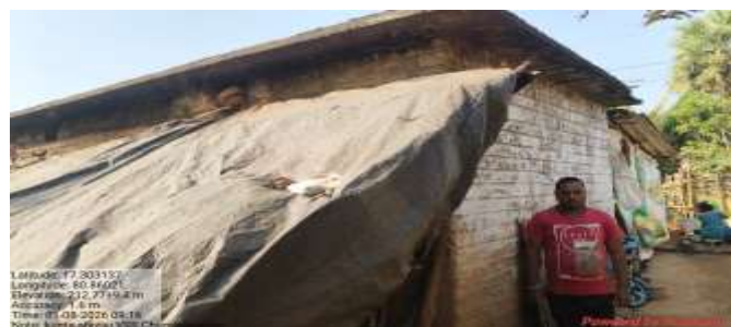
Before House removed
