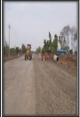
**Remarks -** Proper Barricading of hazard just preceding the railing portion not been done at km 6+200.
