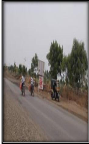
**Remark -** Work-zone sign installed above is not as per IRC standard at km 6+000
