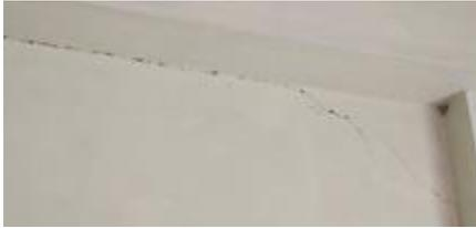
**Fig -3:** Joint Crack
