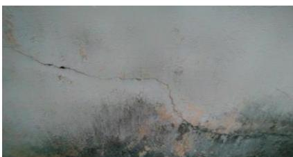
**Fig -4:** Plaster Crack
