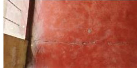
**Fig -5:** Floor Crack
