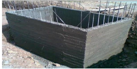
Fig. 2 Underground Water Tank
