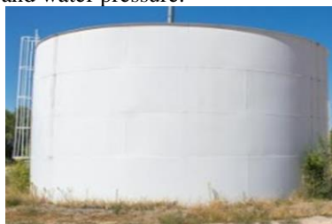
Fig. 1 Water Tank Rest on Ground
