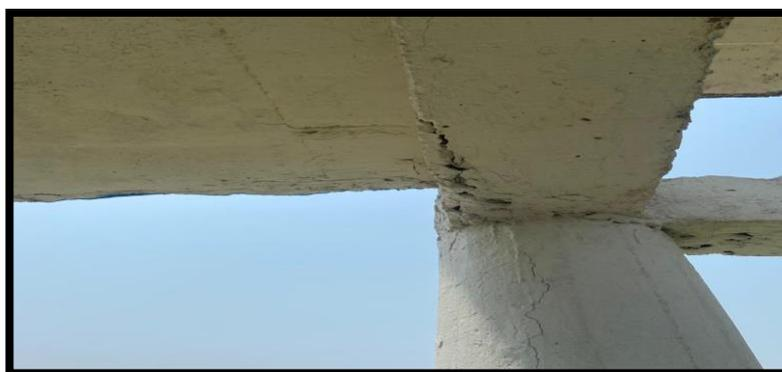
**Figure 17: Shear cracks in the beam**
