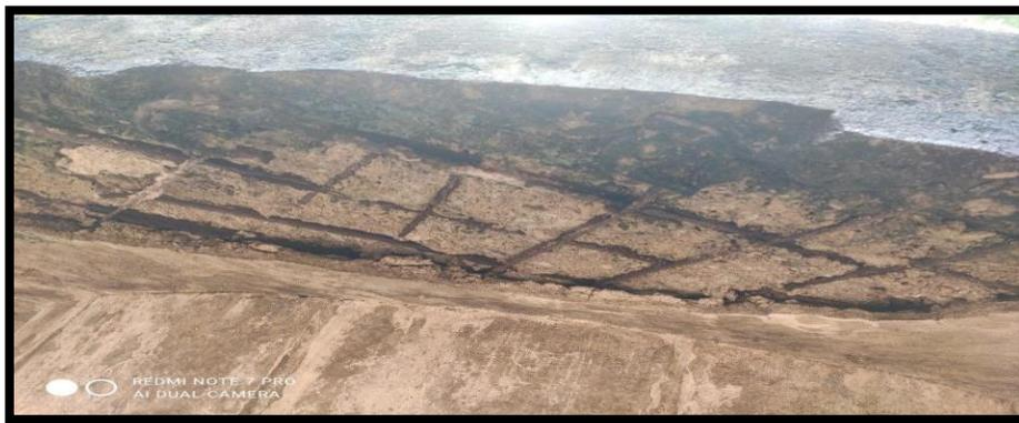
**Figure 11: Slab Plaster Pilling and Reinforcement Corroded**
