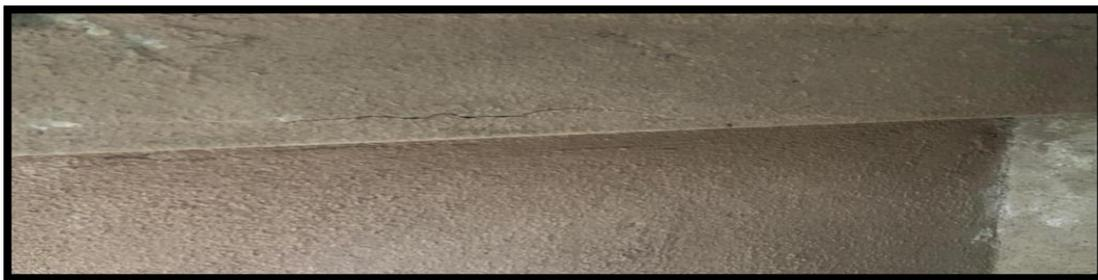
**Figure 10: Flexural Cracks in the Beam**
