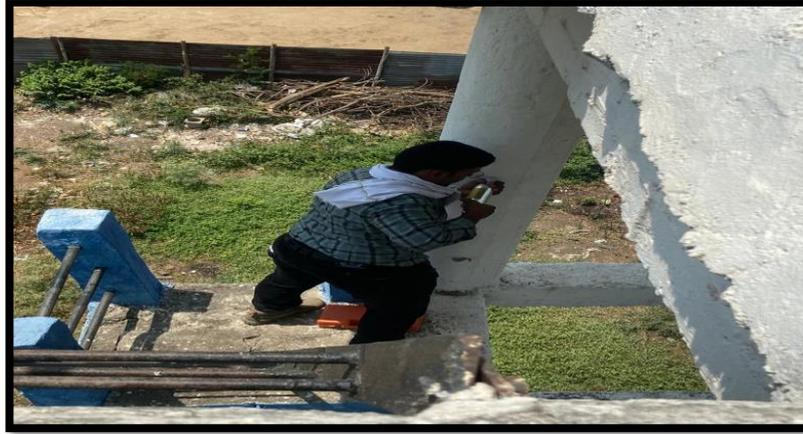
Figure 18: Process of Rebound hammer test
