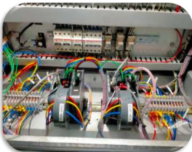
Fig.2 Fixed Power Quality Analyzer Installation
