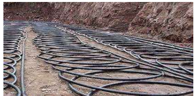
Fig-4: Completed horizontal loop-field trenches prior to backfill
