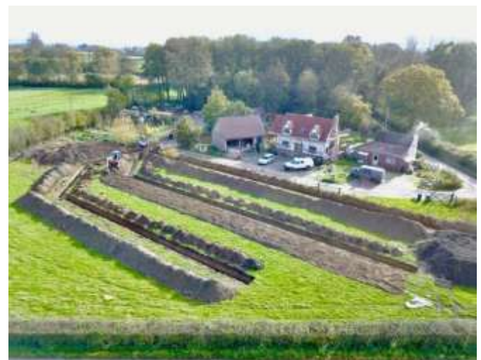
Fig-3: Horizontal ground-loop trenching and pipe-coil installation
