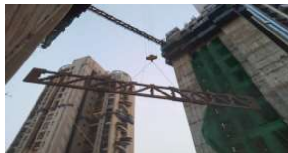
Stage V: Installation and bracing
