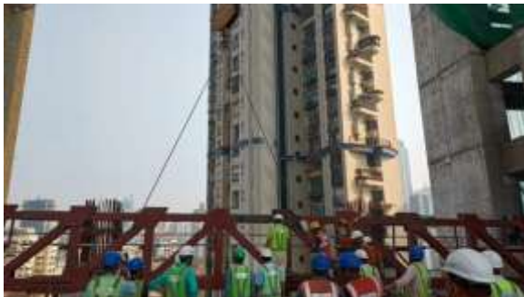
Stage IV: Truss lifting using tower crane
