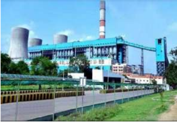
Fig.1. Thermal Power plant Koradi
