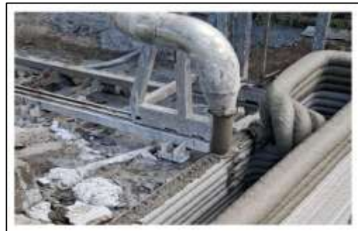
Fig.4. Removal and assembly of printed parts
