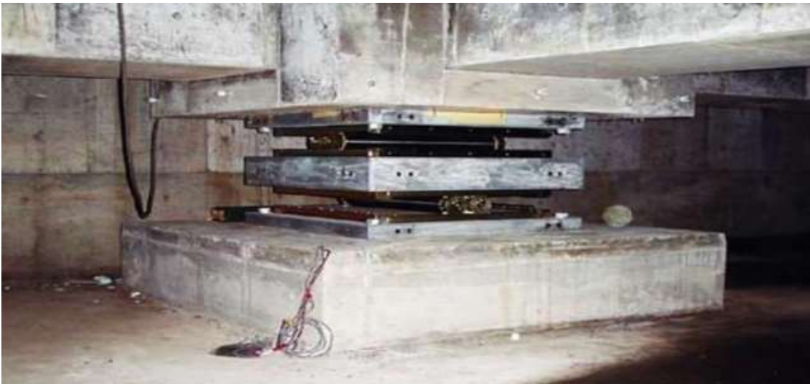
Fig 2. Sliding Base Isolation System
